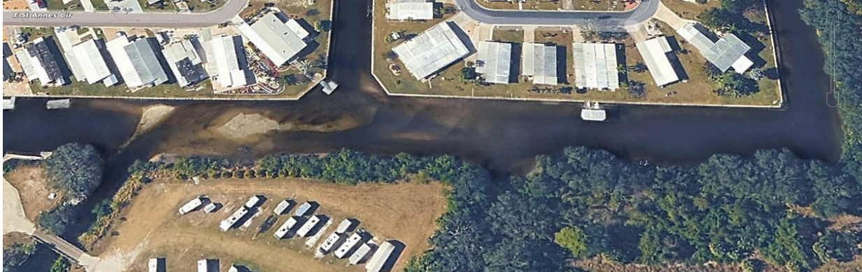
Figure 3 Close Up View of Silt Accumulation in the St. George Canal (2025)
